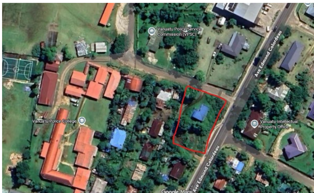
Figure 18 Photos of the site
